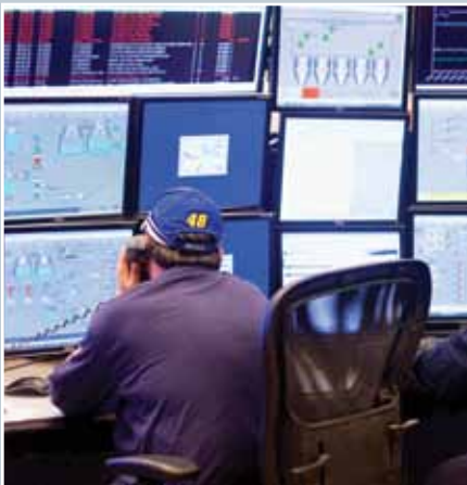
At the Plum Point Energy Station , employees monitor operations of the coal-fired power plant via a bank of computer screens. PHOTO BY SUSAN C. THOMSON
