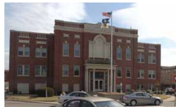
The H.B. Fife Courthouse is the heart of the public square downtown. Elizabethtown and county officials, along with the Chamber of Commerce, are looking at ways to bring businesses back to the downtown area. Motorists traveling through downtown must navigate around the courthouse as they travel on U.S. 31W.
