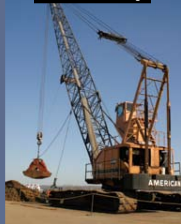
Cranes load and unload goods at the Port of Indiana-Jeffersonville, also known as Clark Maritime Center, along the Ohio River. Clark is the fastest growing port on the Inland Waterway System.
